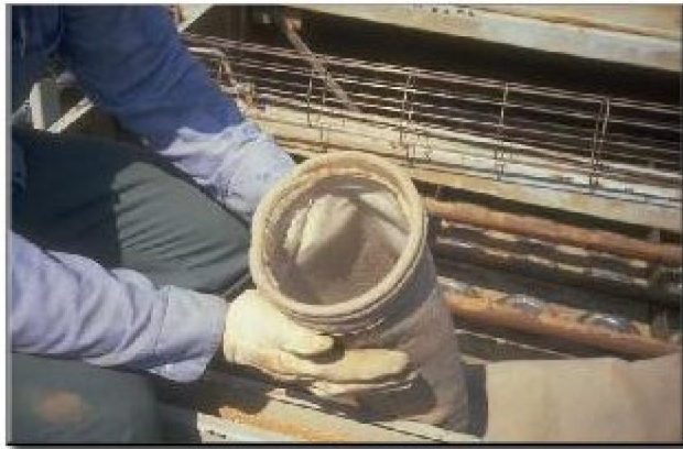
Pulse Jet Baghouse for Particulate Removal
